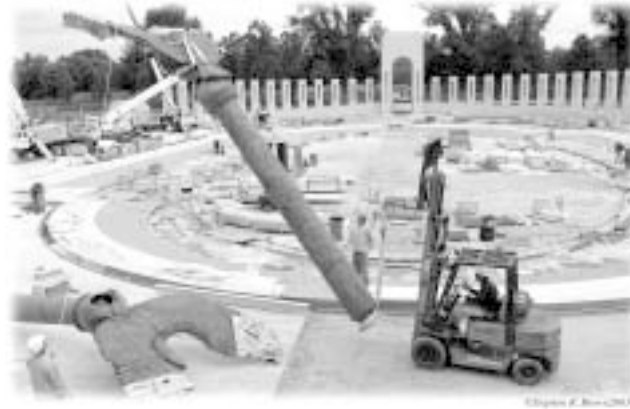
An eagle is lifted into place before being lowered in the Baldachin.
